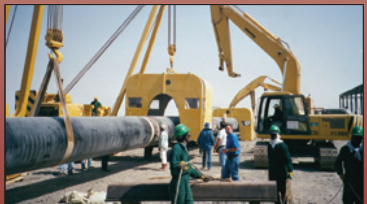
120 cm (48") Wasserpipeline – Hidd-Projekt, Bahrain
